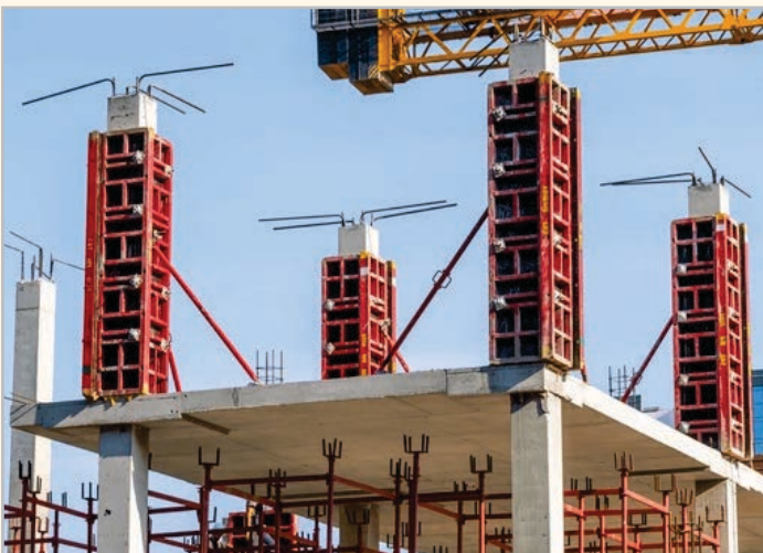
Framework for Concrete Pillars
